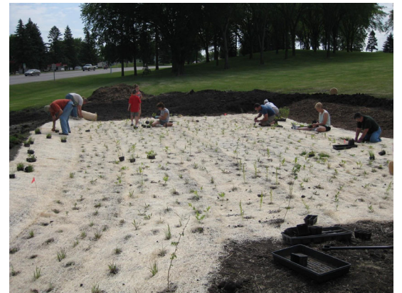
A volunteer crew planted this large rain garden in Fergus Falls in 2009. It captures some of the water from a network of neighborhood storm drains and prevents it from flowing into the Otter Tail River.
