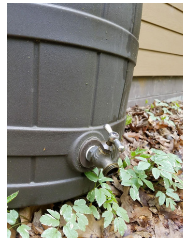
A spigot near the bottom allows you to attach a garden hose to drain the barrel.
